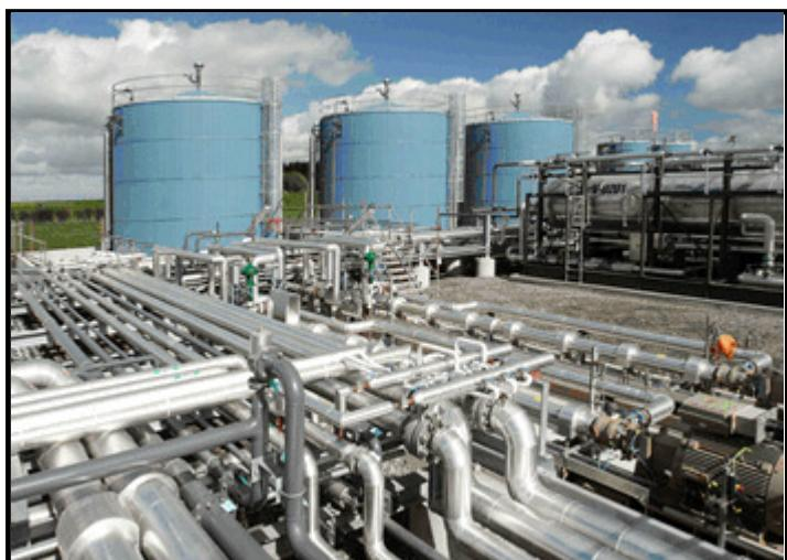
A network of pipes and pumps extracts oil from nearly a mile beneath the surface and carries it through the production process.
